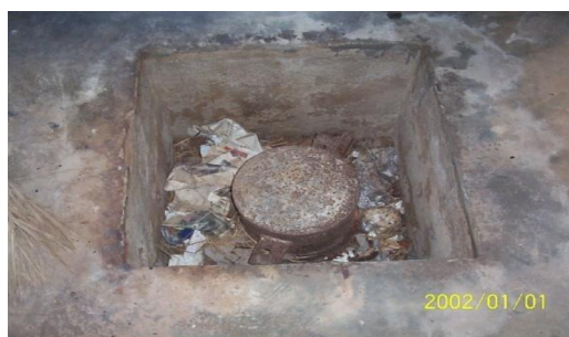
Fig. 17: The Kapasda Water Supply Scheme P.H.No-1, abandoned due to saline water intrusion, Contai, Purba Midnapur.
